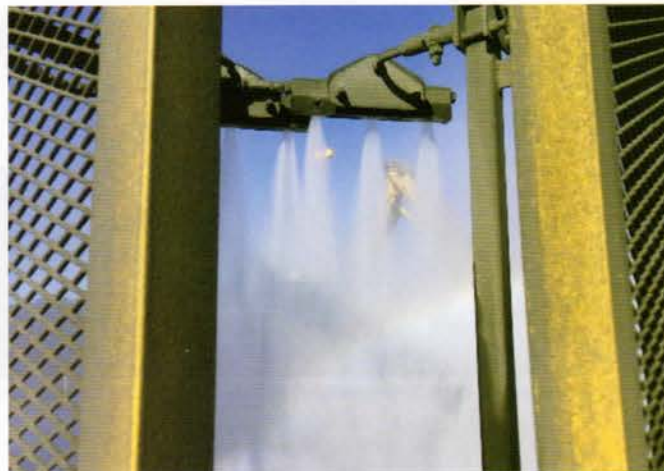
Above: Figure 6: New EnviroMist Dust Suppression System during actual Truck Dumping Operation, showing Micro-Mist Curtain (left) and special Corner Blocks (right).
